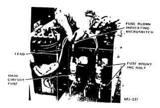
Fig. 17 Main Circuit Fuse (230V, 25A)
