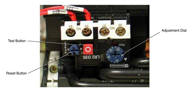
Fig 4.2 Overload Relay Detail
