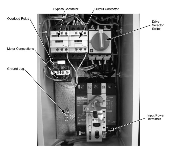
Fig 2.1 Typical Input Power Connection
