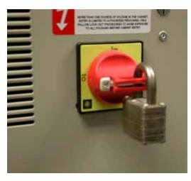
Fig 1.6 Disconnect Handle Positions – Shown OFF, With Padlock
